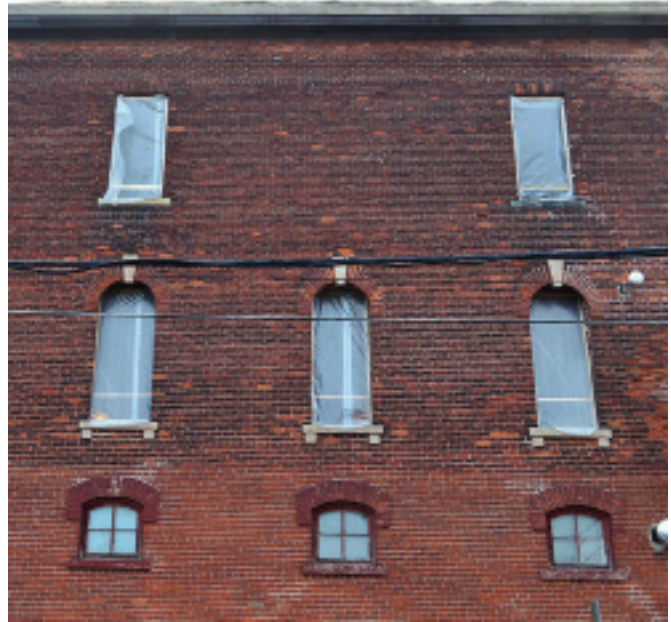
Replacing bricks with original window placement
