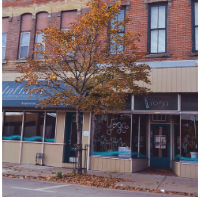
Original door and new door installed that fits guidelines
