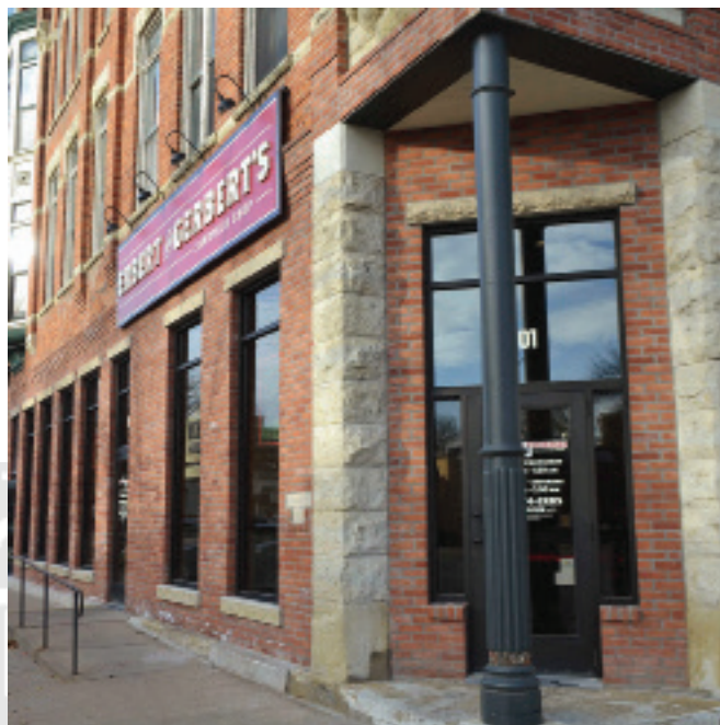
Updated example: Corner repair, windows added, materials replaced on wall
