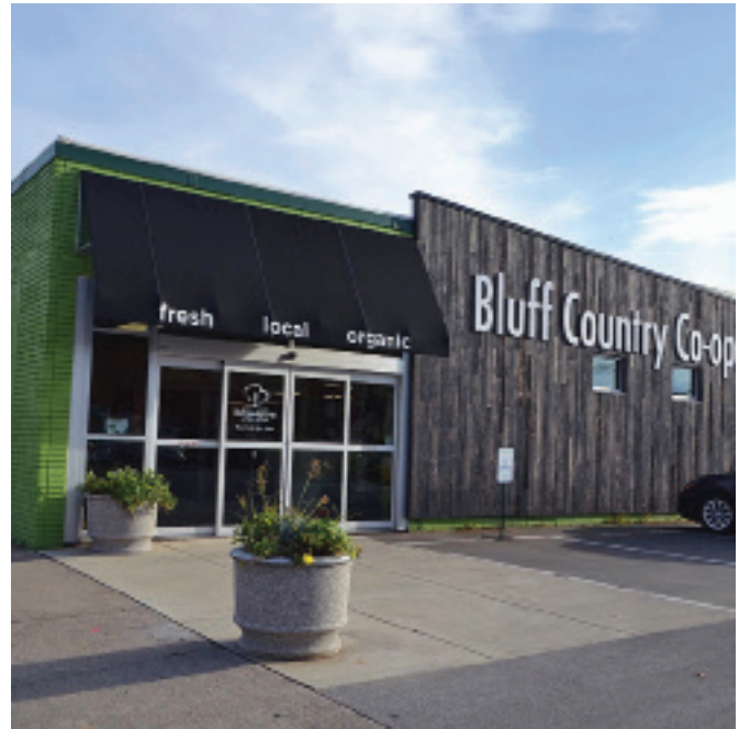
Updated example: Entrance has no steps and proper width
