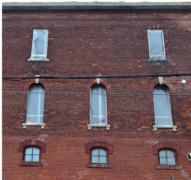
Replacing bricks with original window placement
